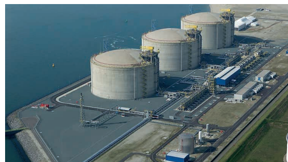
Storage Tanks at Gate Terminal Rotterdam
